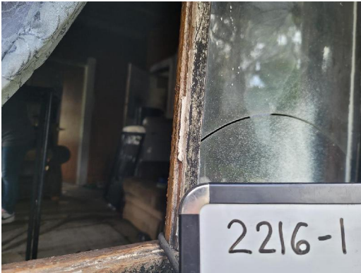
2216-1 Caulk Typical Exterior Windows
