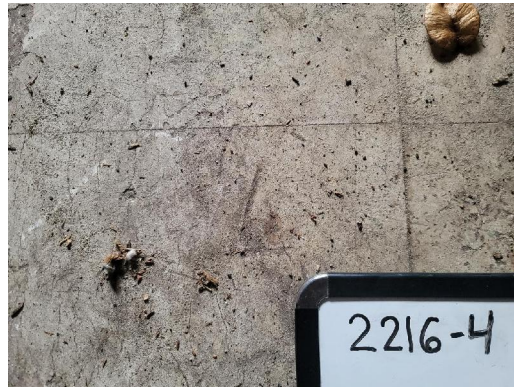
2216-4 12"x12" Floor Tile (2% Chrysotile) Mastic Interior Kitchen/Bathroom (Appx 70 sq ft)
