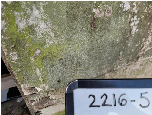
2216-5 Siding Exterior Front Porch Wall
