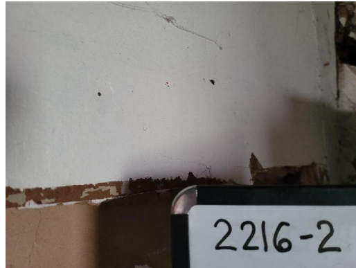
2216-2 Drywall Typical Interior Walls
