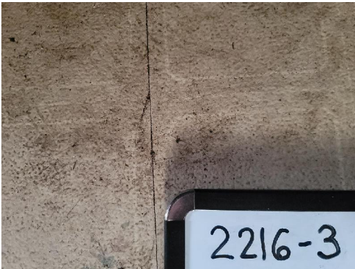
2216-3 12"x12" Floor Tile/Mastic Interior Living Room
